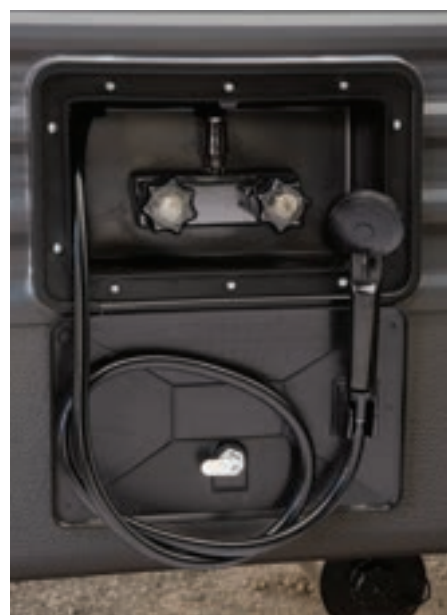
Hot and cold outside shower reduces tracking dirt indoors
